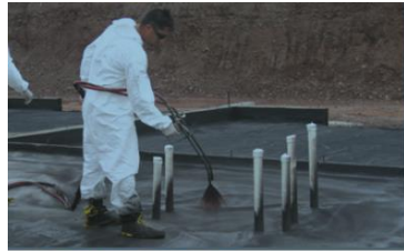
Figure 11. Spraying an emulsified asphalt latex barrier.
